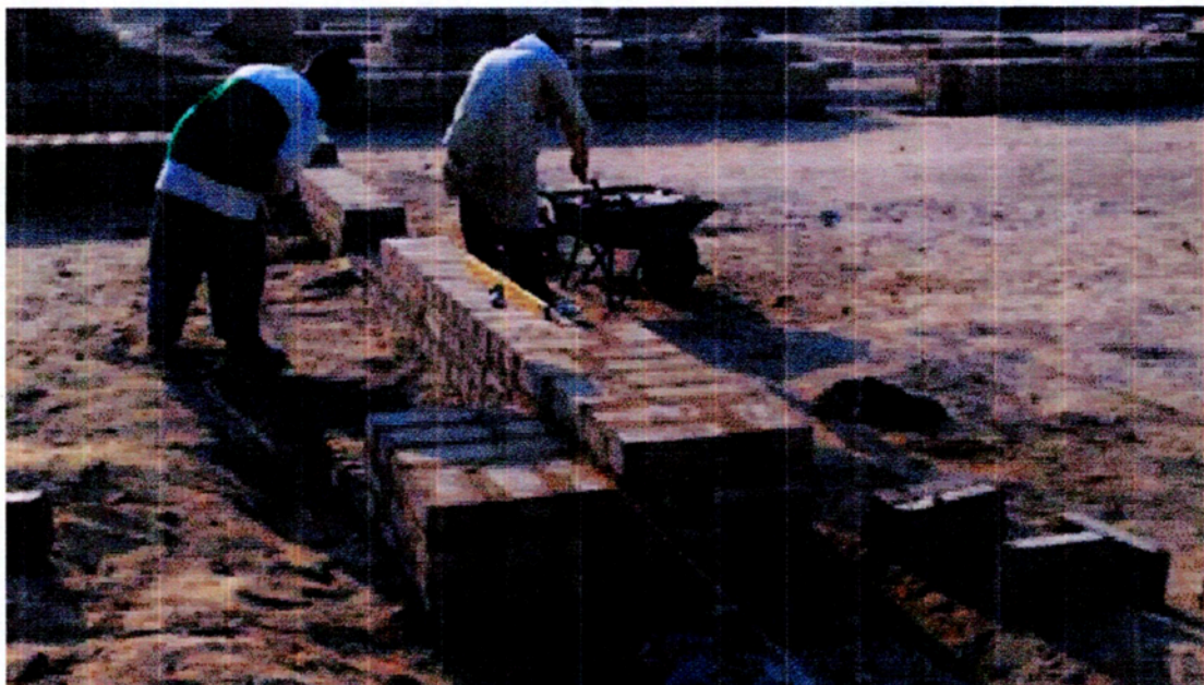
(Mahmoud at work): Local builder Mahmoud Hussein at work, recreating the line of the front wall of the animal building.
